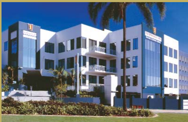
R&D Centre and Head Office, Brisbane
